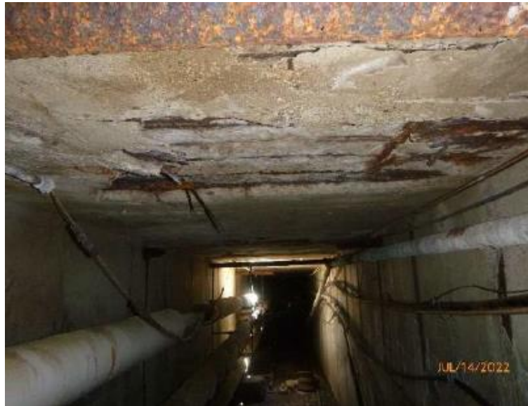
Ceiling deterioration, lots of concrete on floor.
