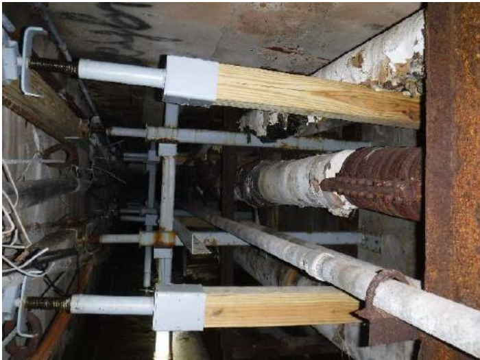
Temporary bracing to shore up walls and ceilings.
