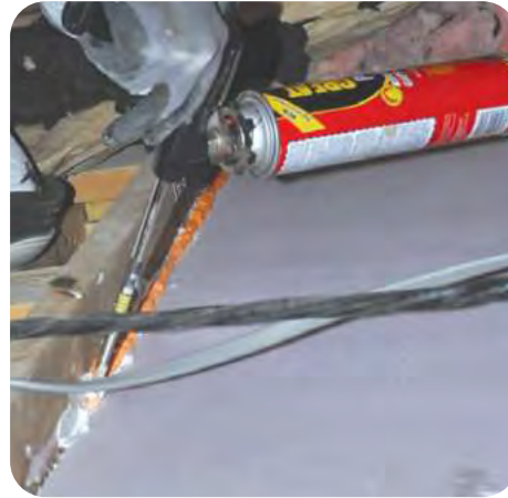
B-2. Seal around infill materials
