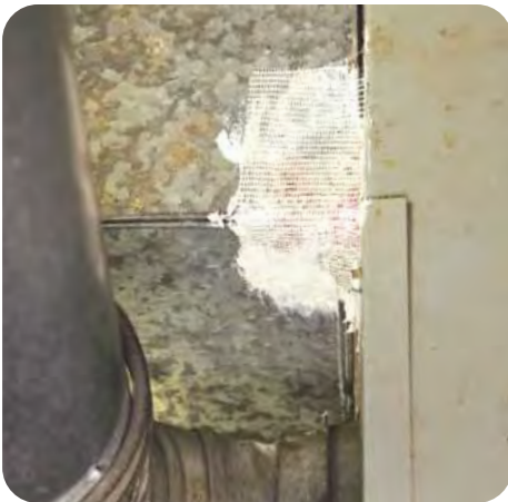
B-4. Push fiberglass mesh into the mastic
