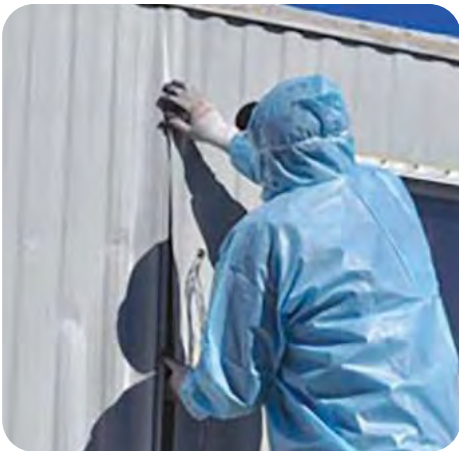
8. Reinstall siding
