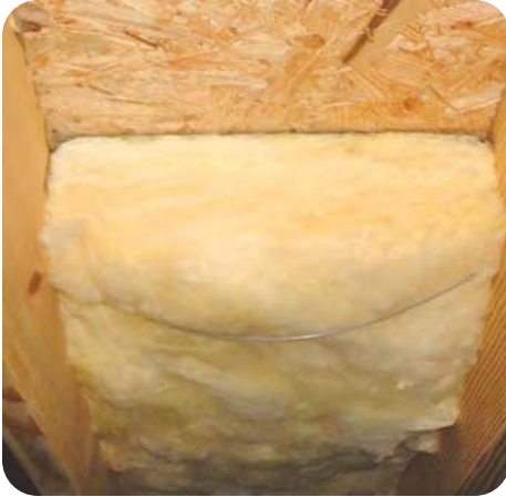
5. Batts are in good contact with subfloor
