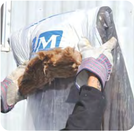
5. Fold batt over end of insulation stuffer
