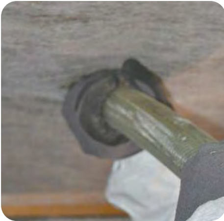
13. Loose fill netting to required density
