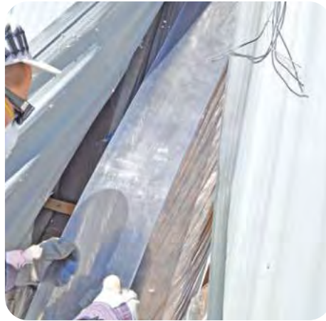
6. Insert batt into cavity, sliding under top belt rail to top of cavity, and ease stuffer back out to allow batt to fill in space
