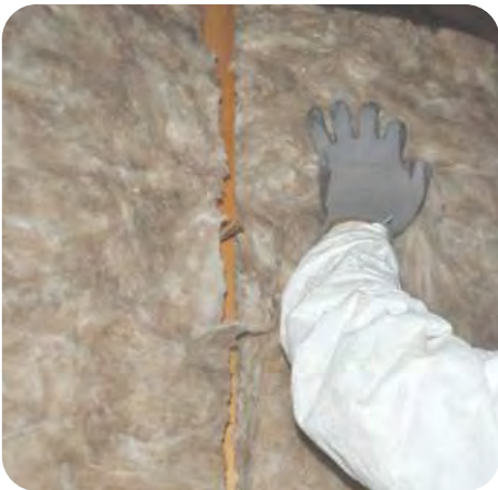
3. Install batts with minimal compression
