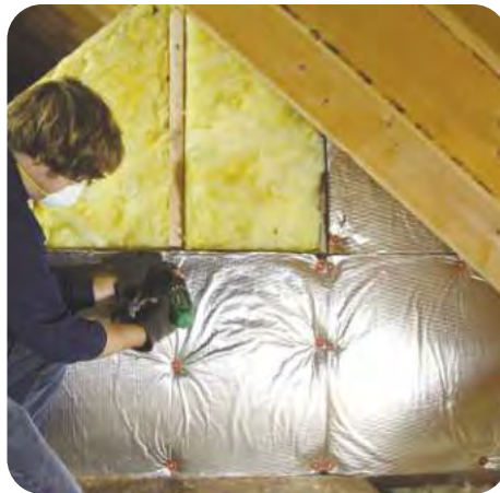
4. Install backing material
