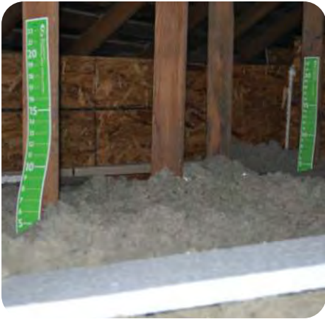
5. Depth rulers installed, 1 per 300 square feet
