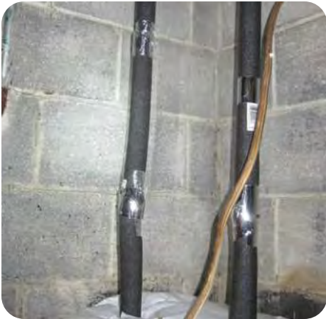
Insulate pipes to a minimum R-3 at least 6 feet from DHW on both hot and cold lines
