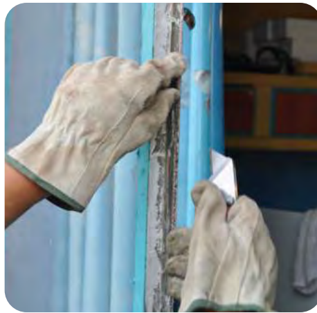
2. Clean all debris, caulk, etc., from sash
