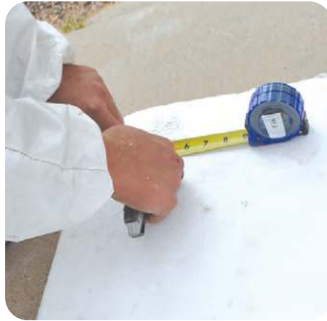
2. Cut blocking material to fit
