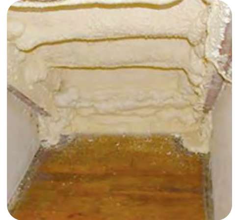
9. Insulate under stairway using insulation indicated by work order
