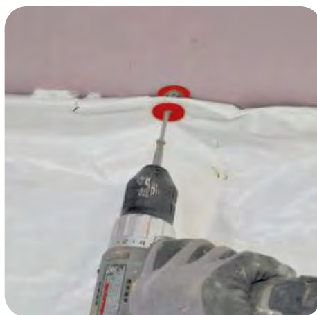
2. Attach new belly wrap
