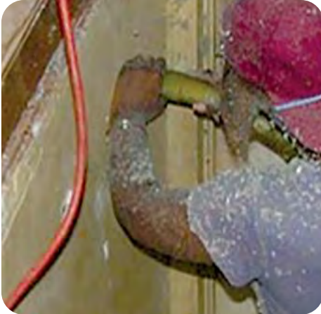
7. Dense pack stairway walls
