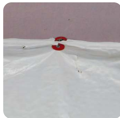
3. Seal seams of belly wrap
