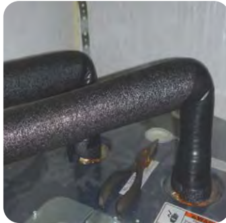
Insulation should be continuous with no gaps
