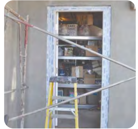
9. Seal rough opening, to prevent both air and water intrusion
