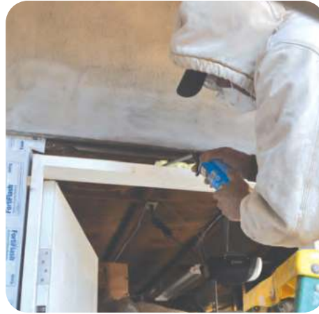
8. Insulate gaps between door jamb and frame
