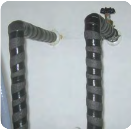
Secure seams with tape
