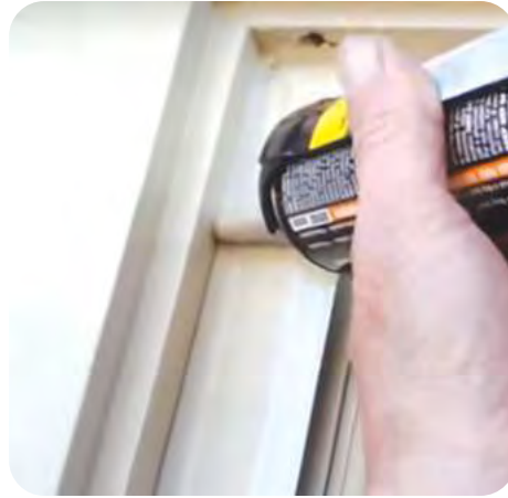
8. Caulk all exterior edges
