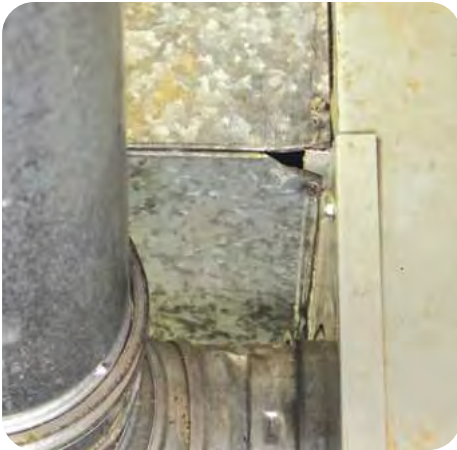
B-1. Small holes and penetrations require one additional step
