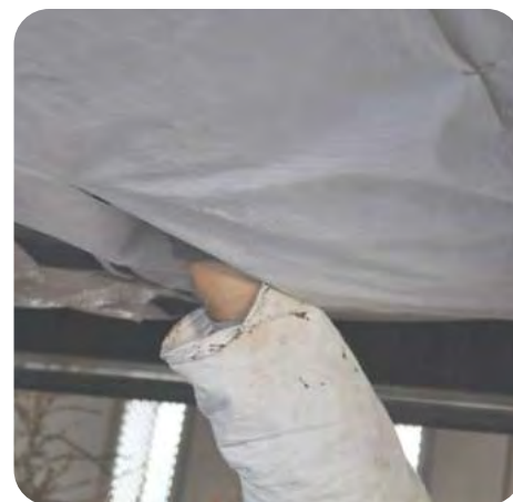
4. Cut access holes to ensure entire cavity will receive continuous and consistent insulation
