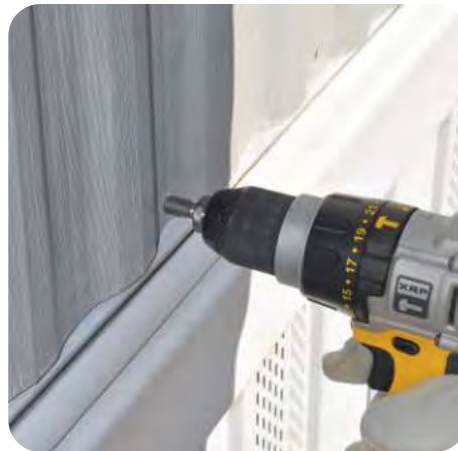
9. Reattach mechanical fasteners
