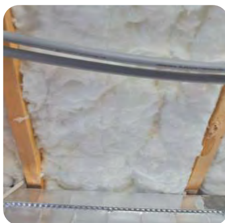
4. Batts installed with no gaps
