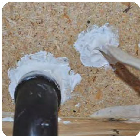
1. Ensure air sealing is complete
