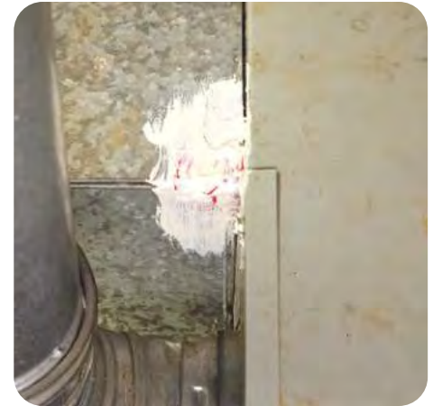
B-3. Apply mastic over the tape
