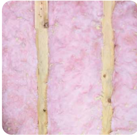
2. Cut batts for exact fit
