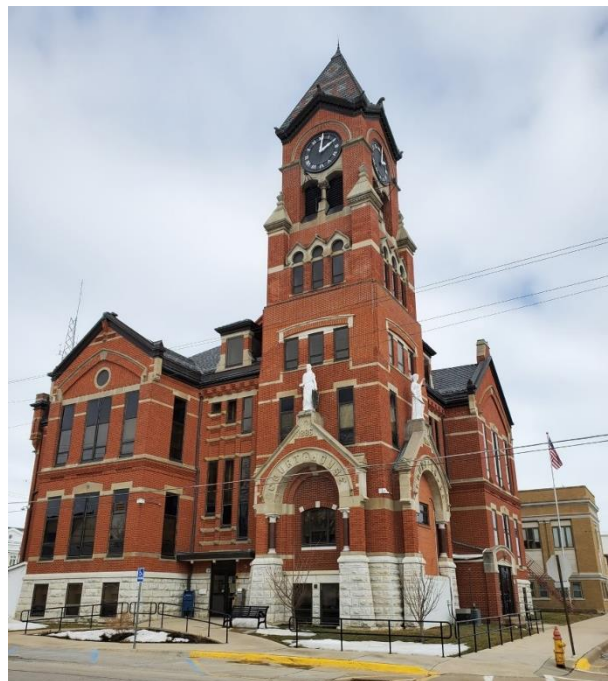
Washington County Courthouse, located in Washington, Iowa.
